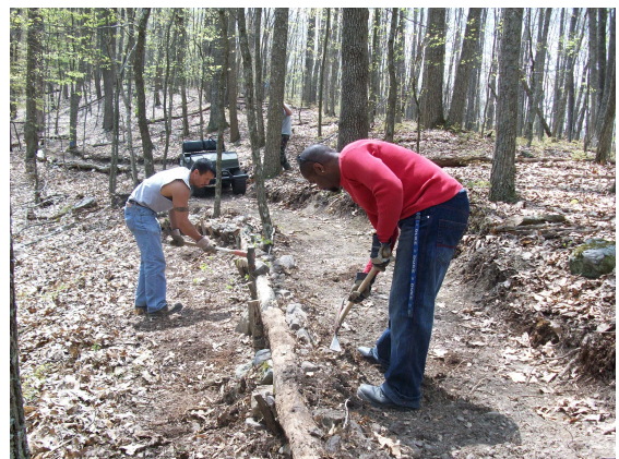
The TRACKS Kids Trail is under construction.
